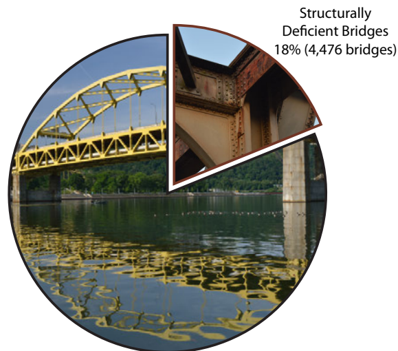
Percent of Structurally Deficient State Bridges source: PennDOT Bridge Management System
